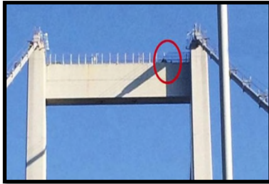
Figure 51 Pro-Erdoğan media used this photo for months to report about a dissenting sniper on top of the tower of the Bosphorus Bridge.
